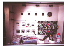
Figure 2.70 Once the vehicles are parked and leveled, the next step is to supply power. With these large production vehicles, you don't simply run a power cord to the nearest Edison socket. Most require a lot of power. An NTSC or PAL analog-equipped 48- to 53-foot trailer usually requires at least 30kW. That's without air conditioning on. Environmental requirements usually kick that consumed power up past 50kW. The newer digitally equipped trucks can increase the needed power by 50 percent (70- to 80kW). The demands of high definition are even higher — over 100kW. Most trucks run on three-phase 208V service. Some are switchable between 220V single-phase or three-phase. Shown is the power panel for a three-phase truck. The forth power cable is for ground. Metering lets the engineer in charge of the truck ensure that voltages are correct before anything in the truck is powered up. Current draw can also be checked here.
