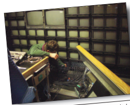
Figure 2.71 Once the side has been expanded out, the right third of the monitor wall in this truck is swung into place and the necessary video feeds are connected.
